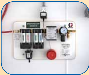
Martech system provides grade D quality breathable air.
